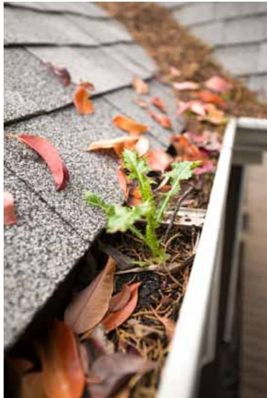
This solutions assumes that your gutter material is of good quality. Aluminum is the most popular material for gutters, but if it's less than .032 inch thick, it's prone to sag – and dent, and crease – no matter what you do.
